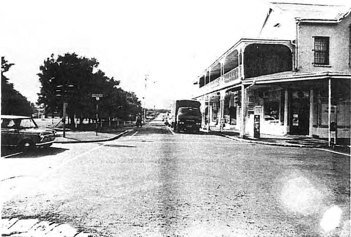
View down Station Road, with the Village Green on the left hand side
